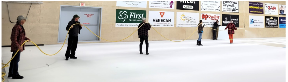
2) A white layer is added using an environmentally friendly chalk like paint. Volunteers are needed to hold up the hose to prevent scratching the previous layer.
